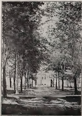
UNION STREET ENTRANCE.
